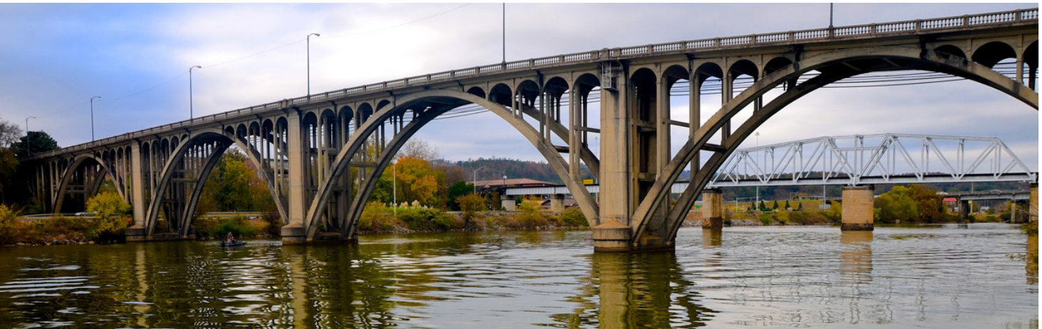
Above: the Coosa River at Gadsden (Source: Glynn Wilson)
