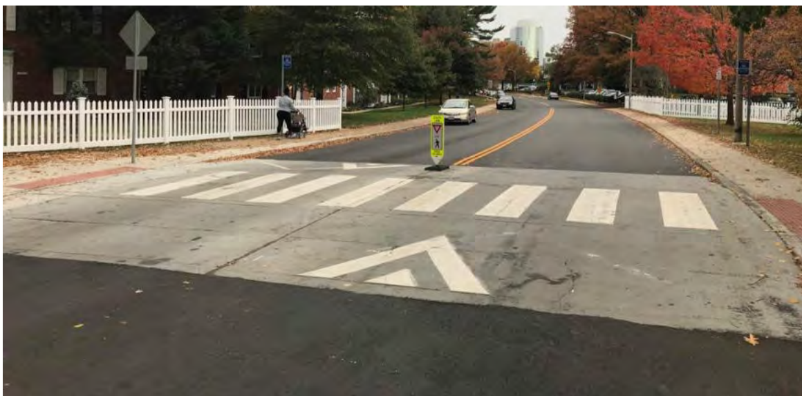
Figure B-24: Example of Raised Crosswalk in Alexandria, VA (Source: PEDSAFE)
