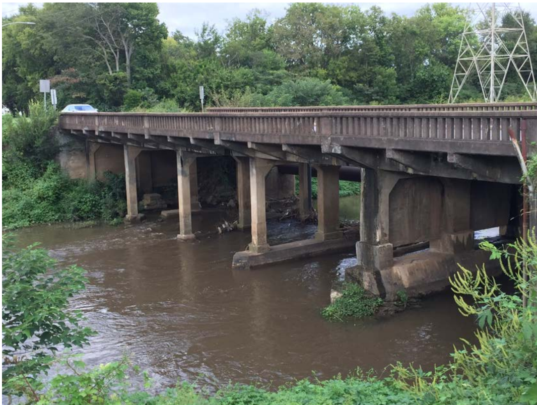
Image 2-3: View of Avenue F Bridge from downstream. Also see Image 1-1, above.
