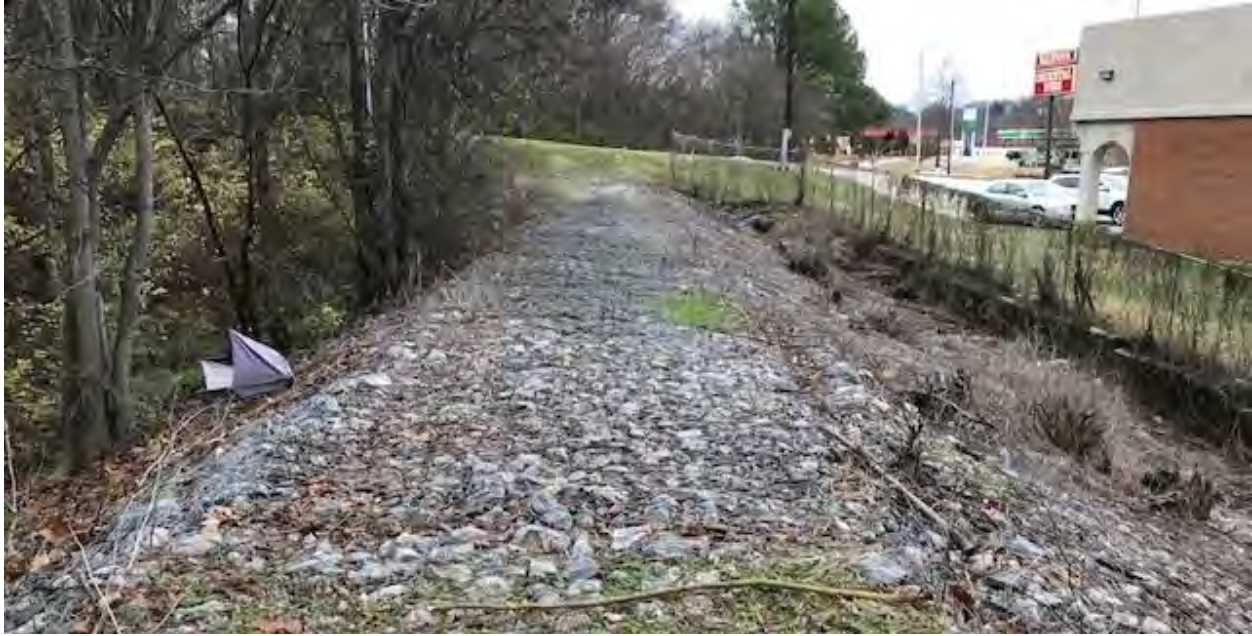
Photo 10: Level path across dam structure near 18th Street South
