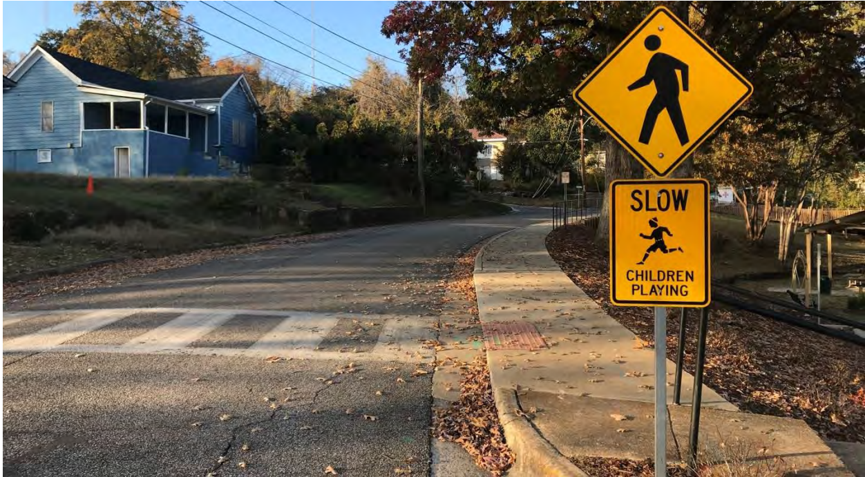
Photo 11: Crosswalk and pedestrian signage on Central Avenue at Spring Park
