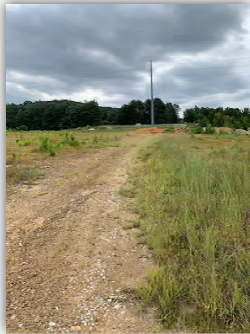
Figure 12: Western Connector Site (View Looking South toward Highway 280)
