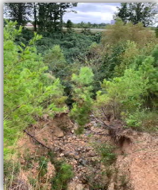
Figure 10: Drainage Ravine (Looking South towards Hwy 280)
