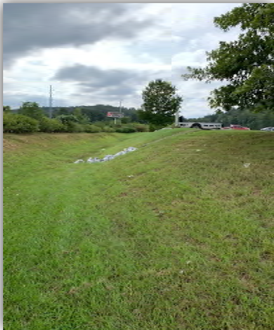
Figure 9: Tractor Supply Drainage Swale (Looking East toward Atchinson Drive)
