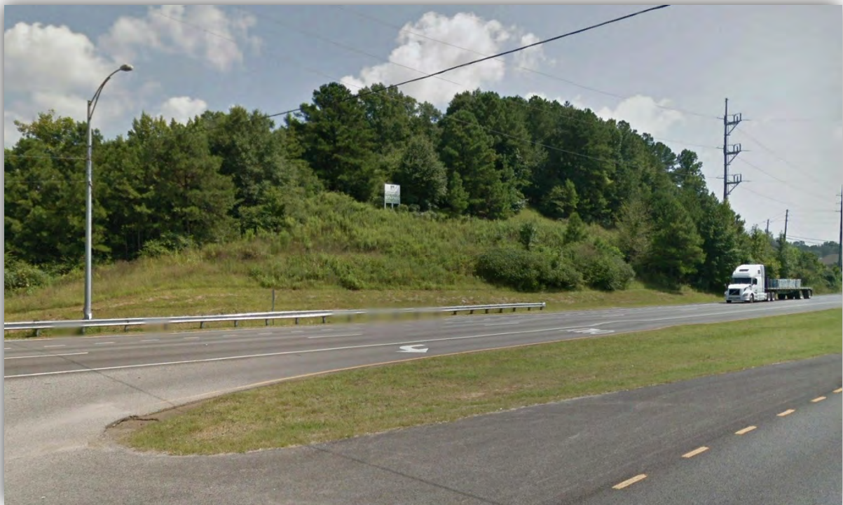
Figure 5: Eastern Connector Rock Cut (North Side of Hwy 280)
