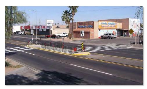
Figure 9: Z-Configuration Crosswalk Design (Source: FHWA)
