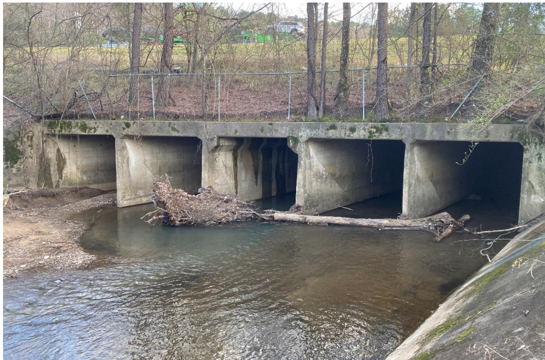
Photo 7: Shades Creek Culvert under Interstate 20
