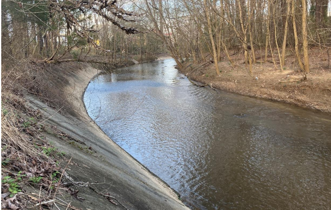
Photo 6: Typical View of Shades Creek within Section C
