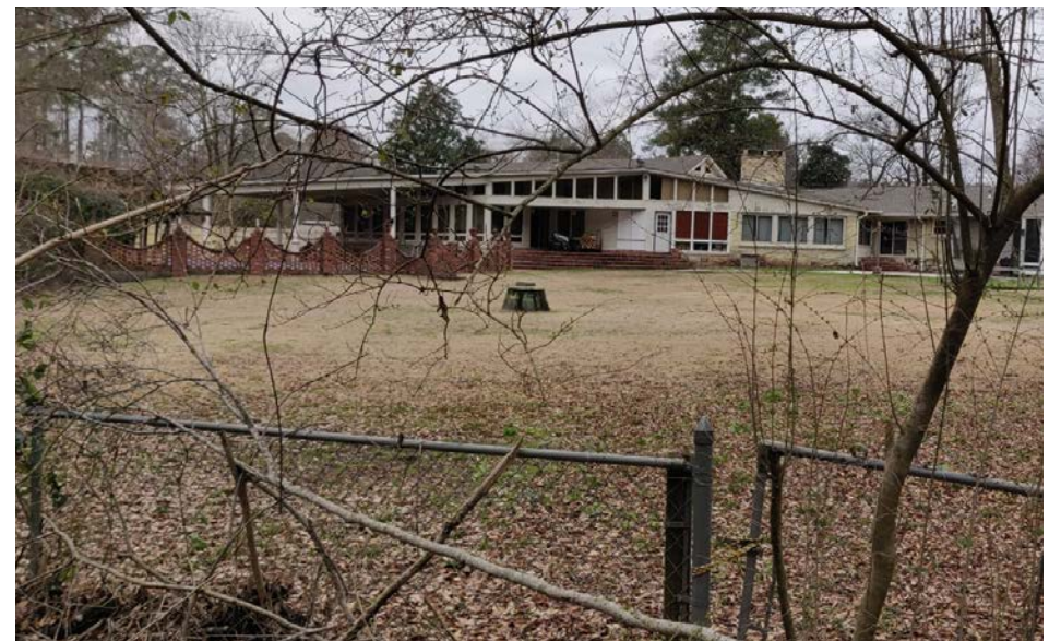
There are a few occurrences of private fences encroaching onto City of Birmingham land and the sewer easement. A full corridor survey is recommended to full assess the extent of these encroachments.
