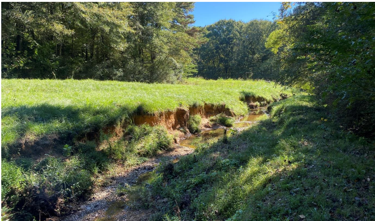
Photo 19: View of the Drainage Channel Separating Sections C and D
