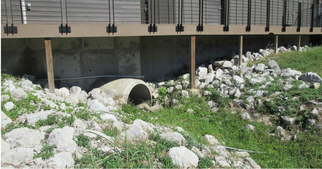
Photo 11: Drainage Pipe under Trussville Entertainment District Stage
