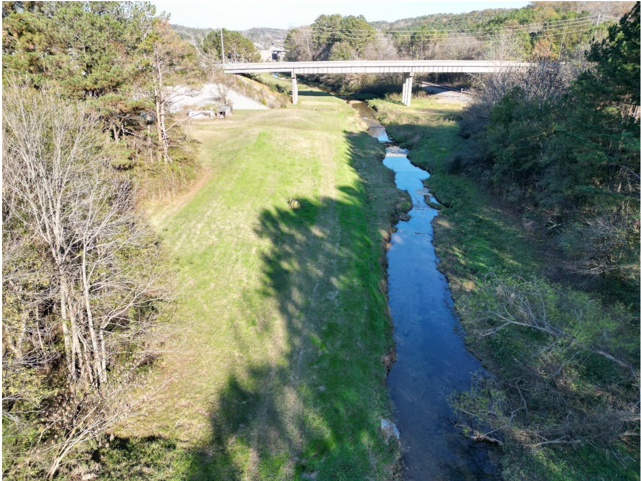
Photo 26: Overhead View of the USACOE-Jefferson County Easement
