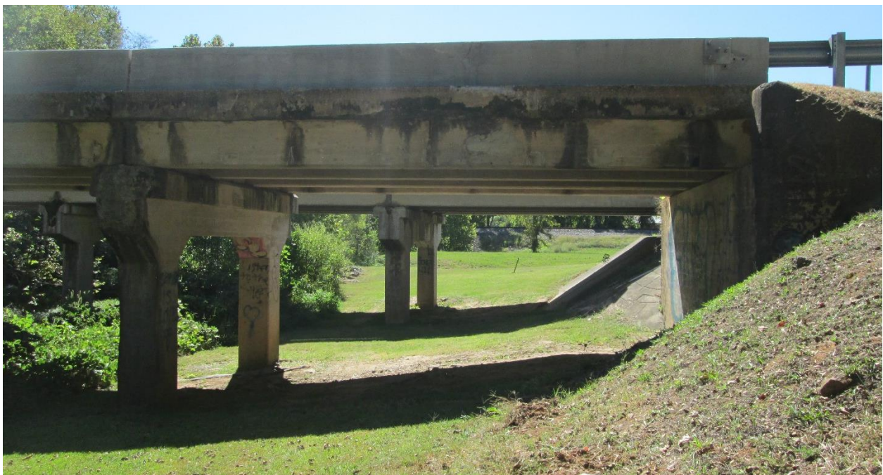
Photo 6: View of US-11 bridge over the Cahaba River (Potential Trail Location)
