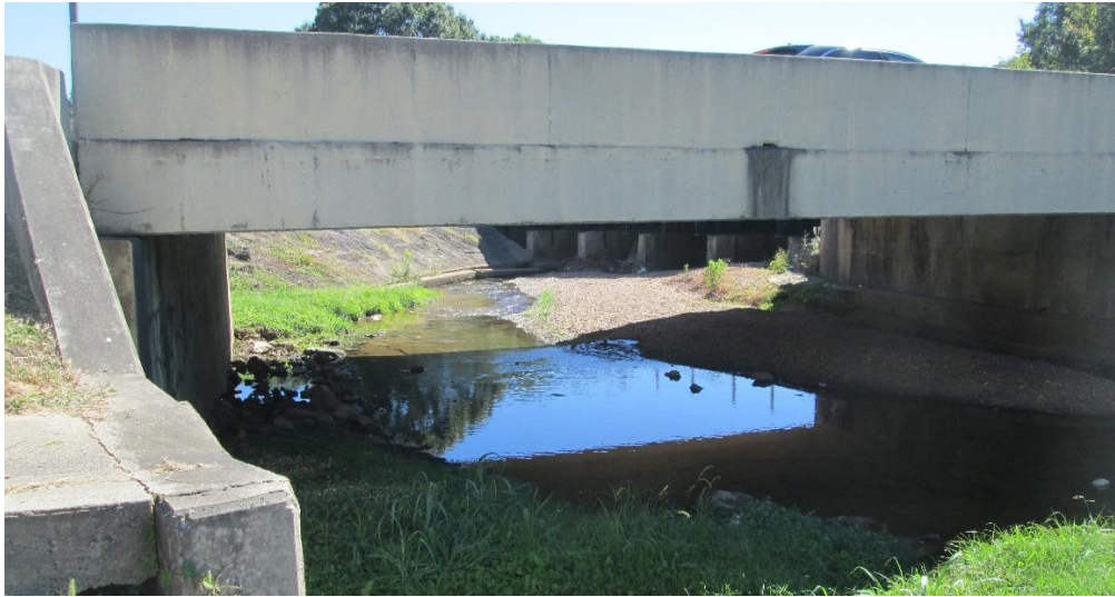
Photo 7: Pinchgut Creek under Chalkville Road
