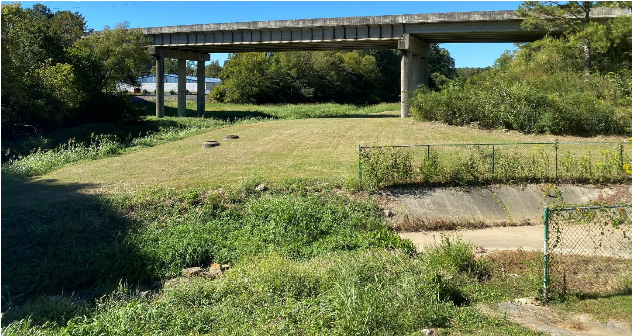
Photo 14: Drainage Channel Terminus at Pinchgut Creek
