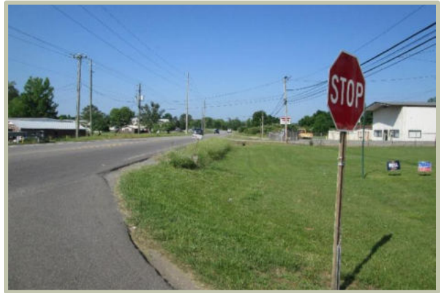
Photo 8: Looking Southbound along US-411 from Avalon Drive
