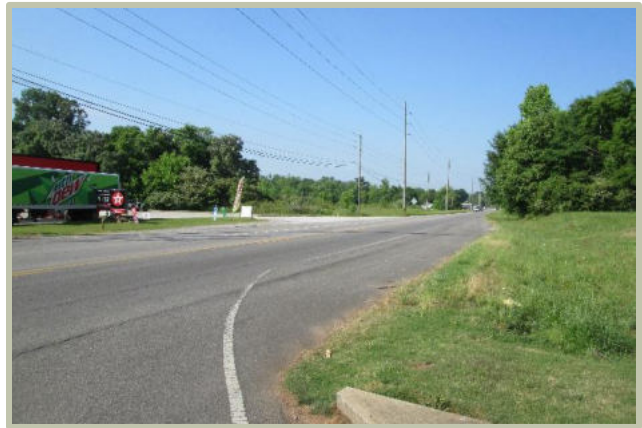
Photo 4: Looking Southbound along US-411 from Washington Drive
