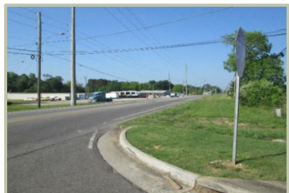
Photo 2: Looking Southbound along US-411 from Avalon Drive
