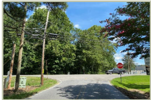
Photo 22: Stuart Drive Approach to US-411
