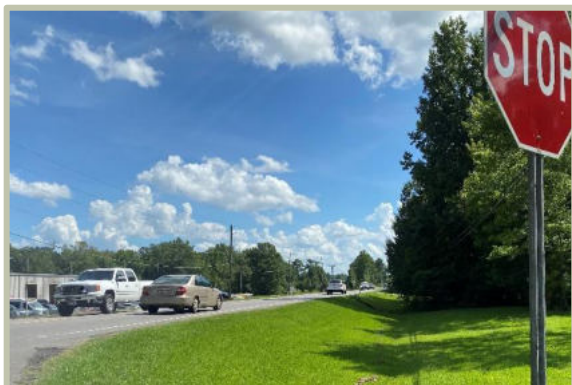
Photo 23: Looking Southbound along US-411 from Stuart Drive
