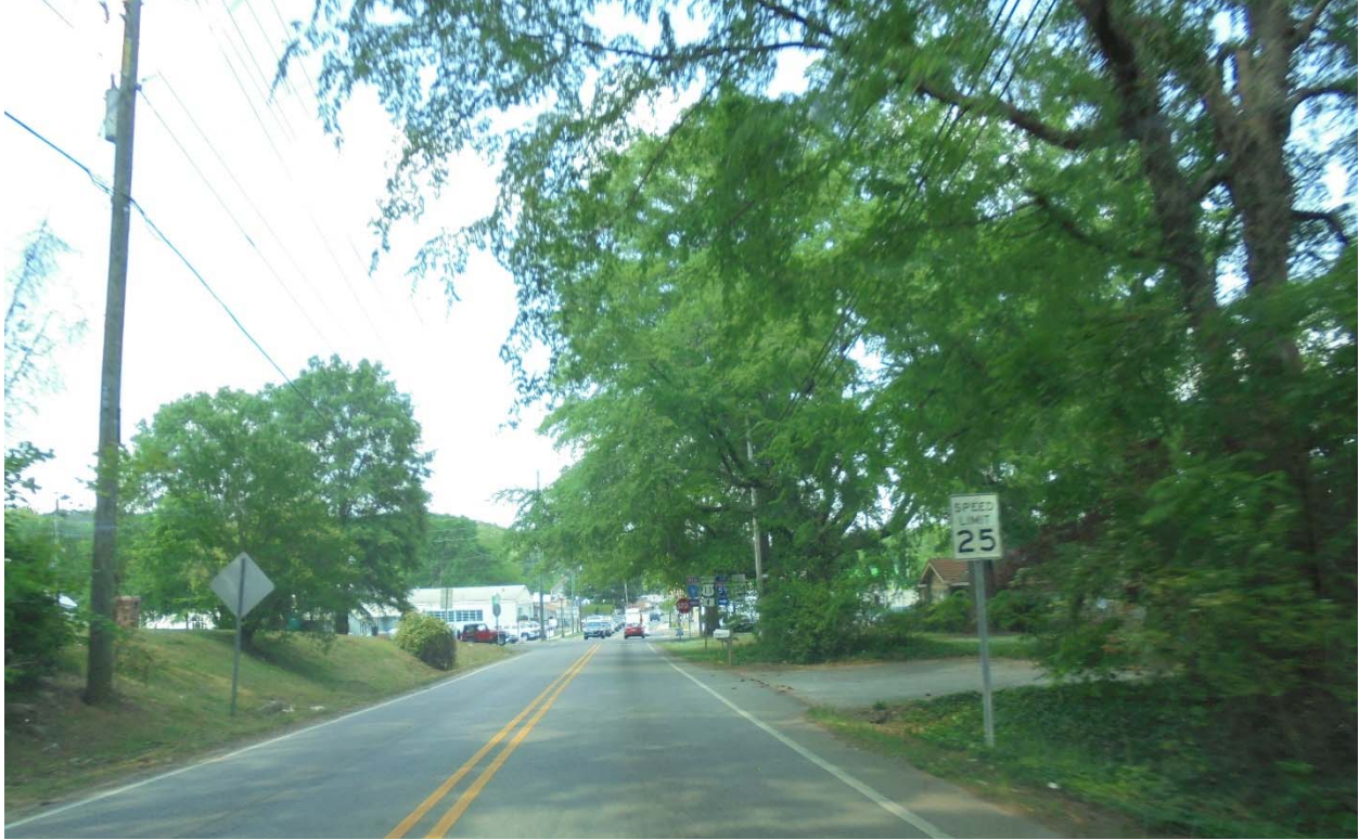
U.S. Highway 11 (Main Street) Northbound approaching State Route 174
